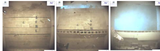
Unprotected Walls Can Collapse and Send Dangerous Debris into Building
